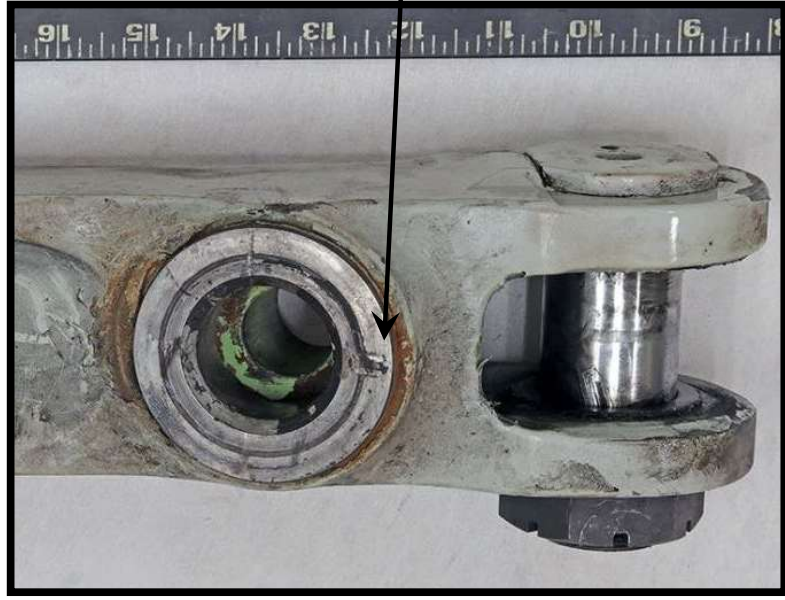
Figure 78. Detailed view of Lower Drag Strut (AFT Side).
